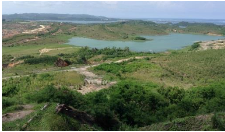
Figure 13. Tubig Sanlay Water Catchment
