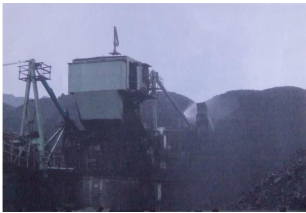
Figure 4. Water sprinkle in the coal blending stockpile
